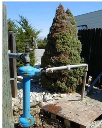
**Figure 1:** The wellhead on your property will typically include a pipe leading to your pressure tank.
